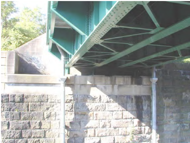
Photo No.4 South Abutment (near) - Elevation
