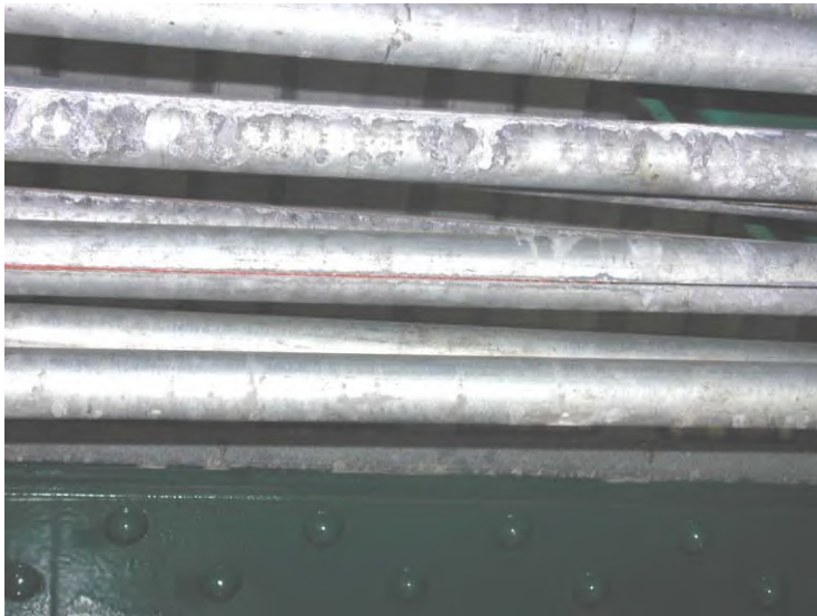
Photo No. 12 Conduit, Span 1 – note longitudinal crack/split
