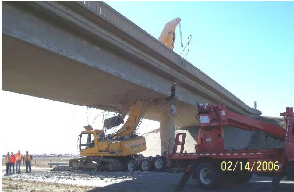
Figure 4.4.2 Accident Involving Construction Equipment and a Bridge
