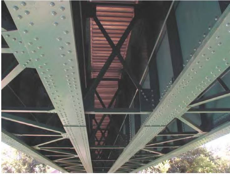
Photo No.9 General Underside View – Span 2
