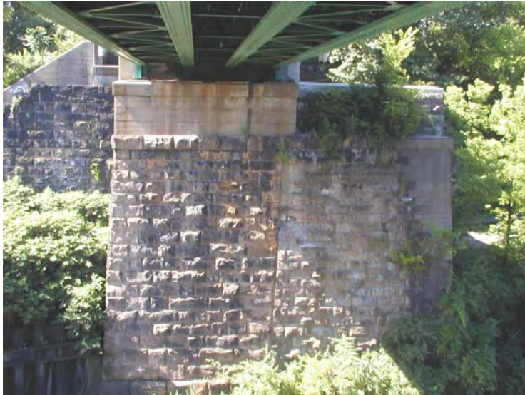
Photo No.6 Pier 1 - North Face (Looking South)
