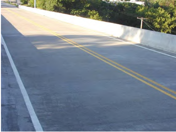
Photo No. 11 General Deck View
