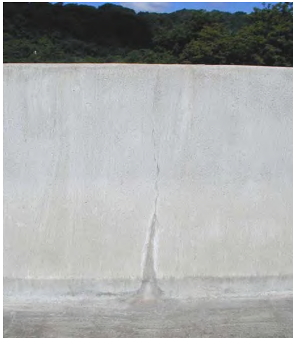
Photo No.16 Typical parapet crack
