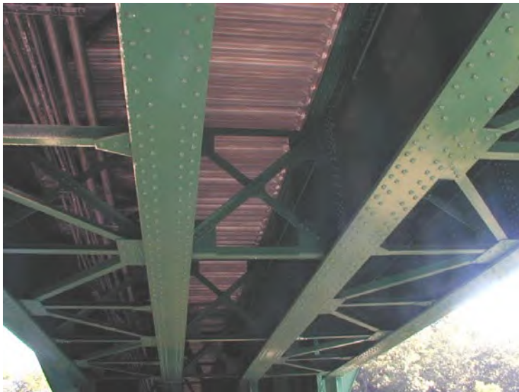
Photo No.8 General Underside View - Span 1
