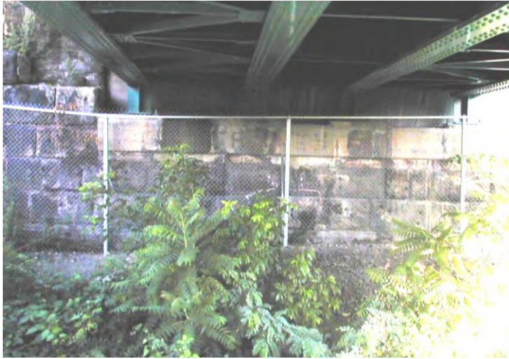
Photo No.5 North Abutment (far) - Elevation
