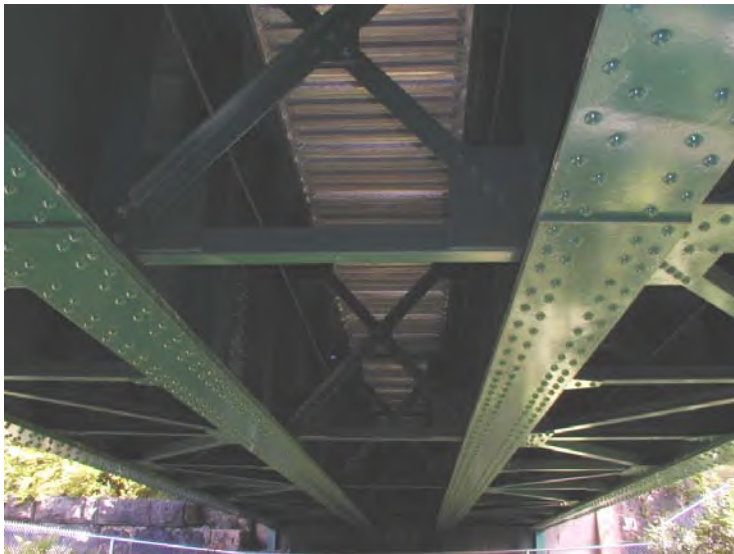
Photo No. 10 General Underside View – Span 3
