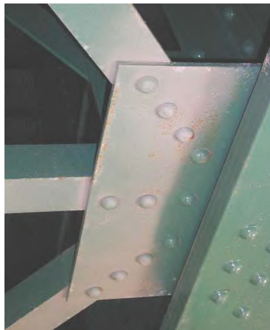
Photo No.18 Lateral bracing connection between beam #3 and #4, in span 2 – note no final paint coat, and rust freckles
