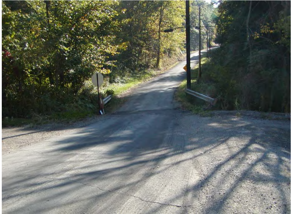
Figure 4.6.1 Near Approach - Toward Bridge
