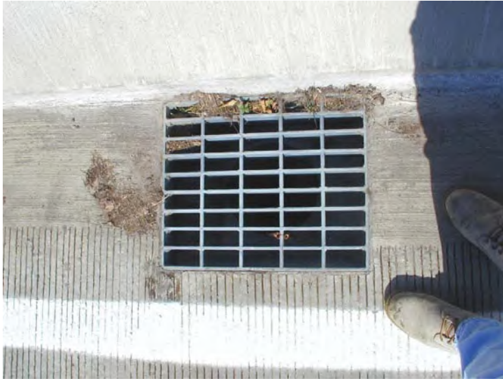
Photo No. 15 Typical PennDOT Type 1 Scupper
